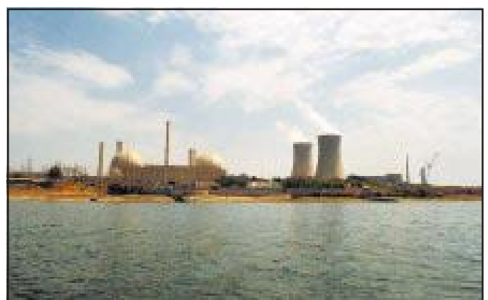
Rajasthan Atomic Power Project
