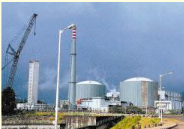
Kaiga Atomic Power Project
