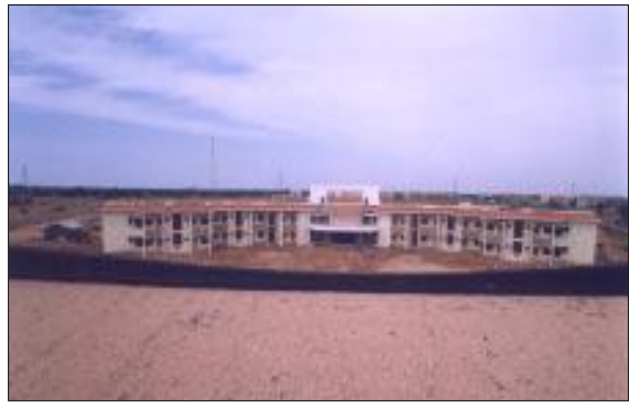
SRI Guest House nearing completion.
