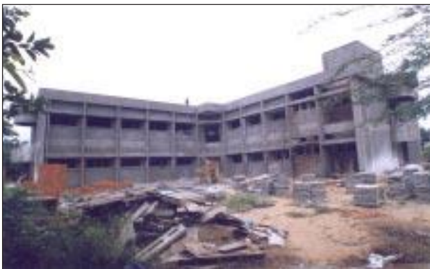
SRI building under construction.
