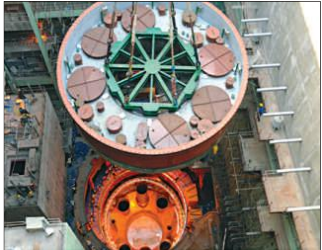
Placing of roof slab in the reactor vault for alignment checking
