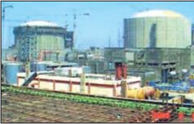
TAPP 3&4 under Construction
