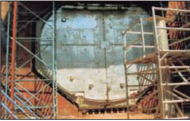
End shield installed in Calandria Vault of KGS 3
