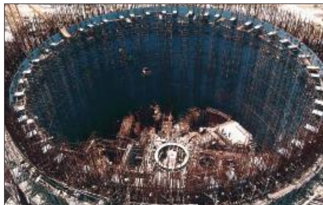
A view of KK-NPP Unit-1 under construction
