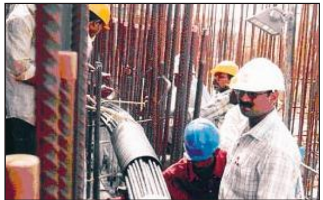
KK-NPP Pre-Stressing System Mock Up for Strand Threading
