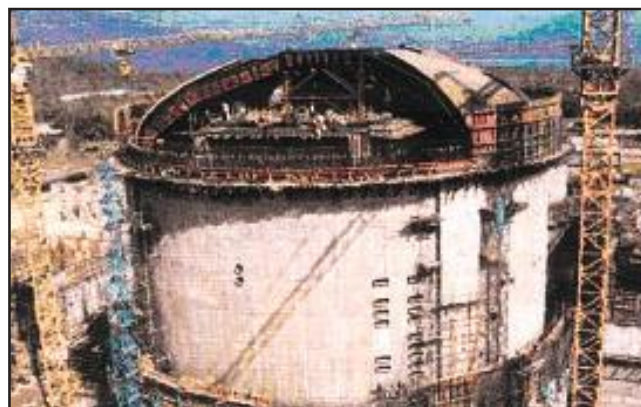
KGS3: Reactor Building
