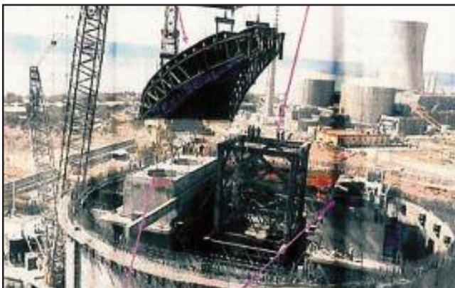
RAPP-5: Installation of Dome Truss
