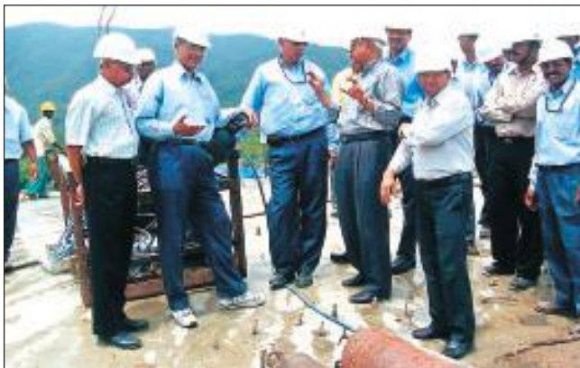
CESSC visiting dome construction of Kaiga-3&4
