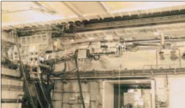
TAPP-3: Testing of Fueling Machine on Rehearsal Facility
