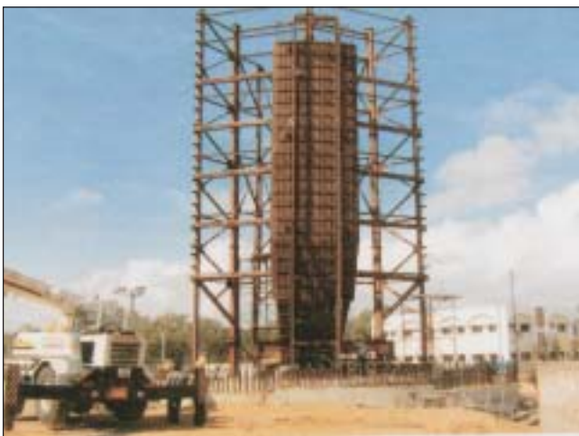
PFBR: Mock-up for Construction of Reactor Vault
