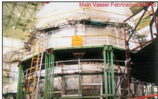
Main Vessel Fabrication at Site Assembly Shop of PFBR
