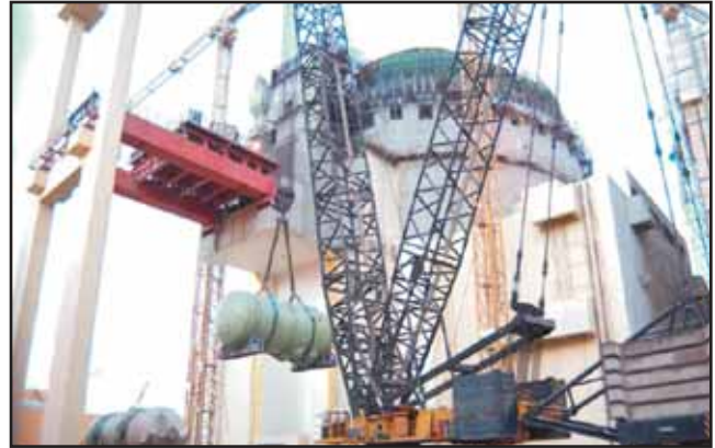
KK-NPP Unit-1: Reactor Pressure Vessel being taken inside Reactor Building
