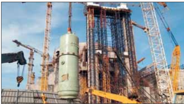
Erection of Pressurizer of Unit-2 of KK-NPP in Progress
