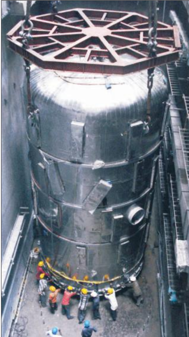
PFBR Argon Buffer Tank (ABT) being lowered into ABT cell
