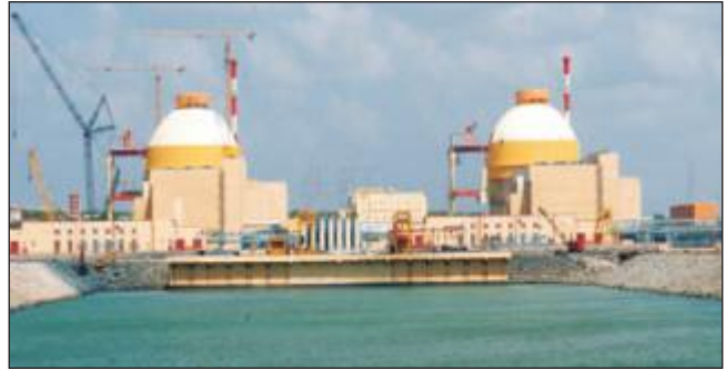
Kudankulam Nuclear Power Project (KKNPP) Units-1&2
