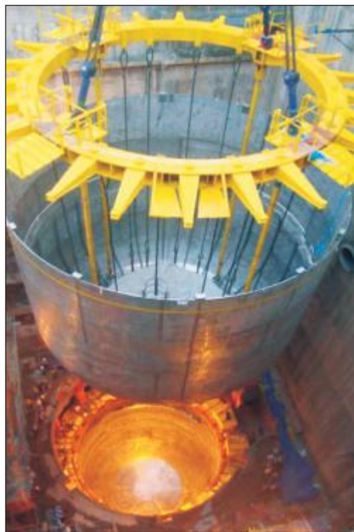
PFBR Main Vessel being Lowered into Safety Vessel
