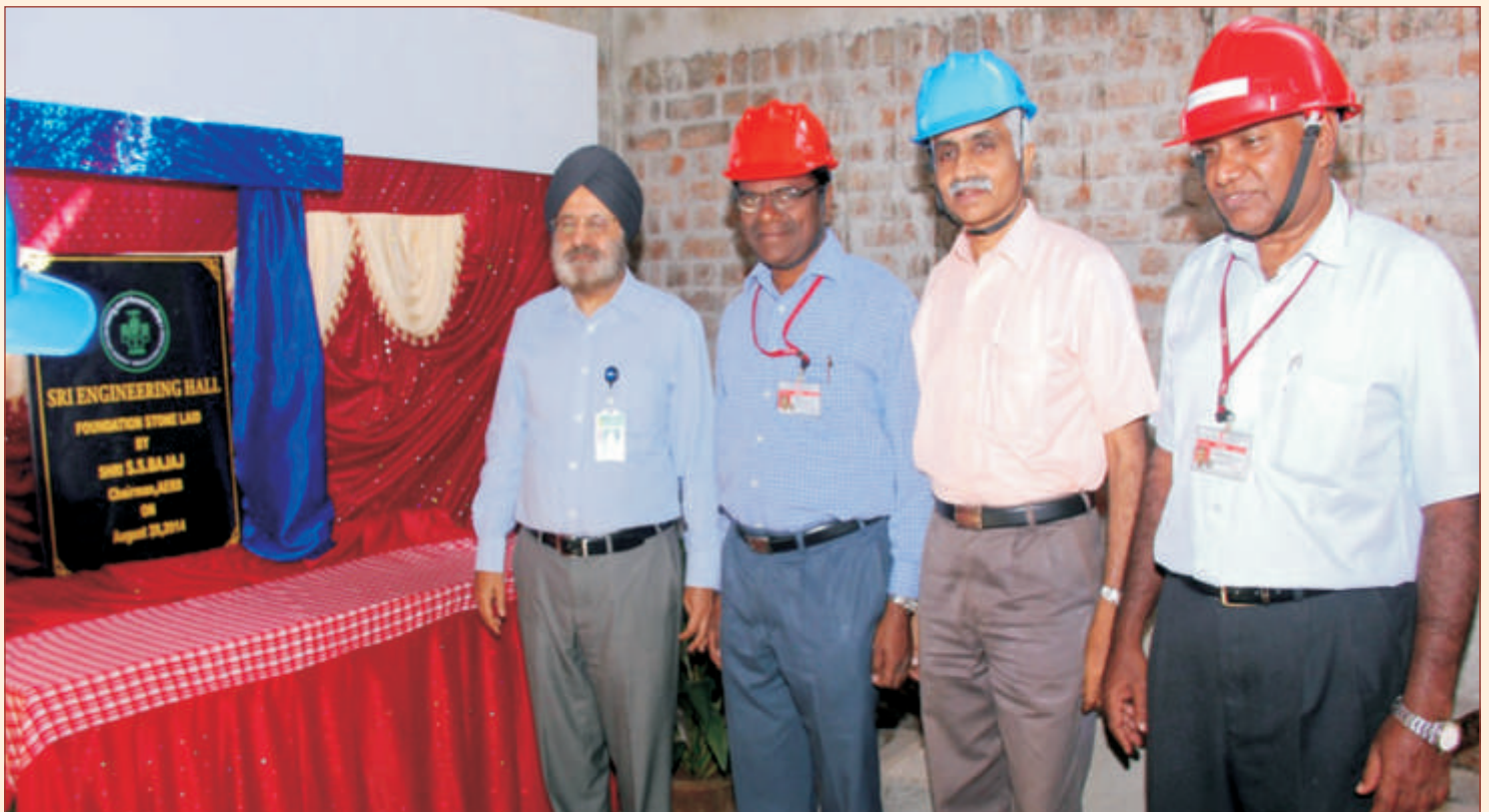
Shri S.S. Bajaj, Chairman AERB along with Shri C. Sivathanu Pillai (AD, CEG), Shri V. Balasubramaniyan (Dir. SRI) and Shri B. Hari Krishnan (Head, CWMD, CEG) during the unveiling ceremony of the Plaque in the SRI Engineering Hall under construction.
