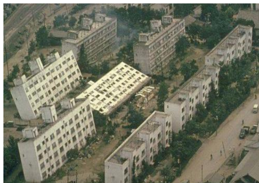
Figure 14 - Adverse effects of liquefaction during Nigata earthquake 1964 [Source: Wikipedia(W1)]
