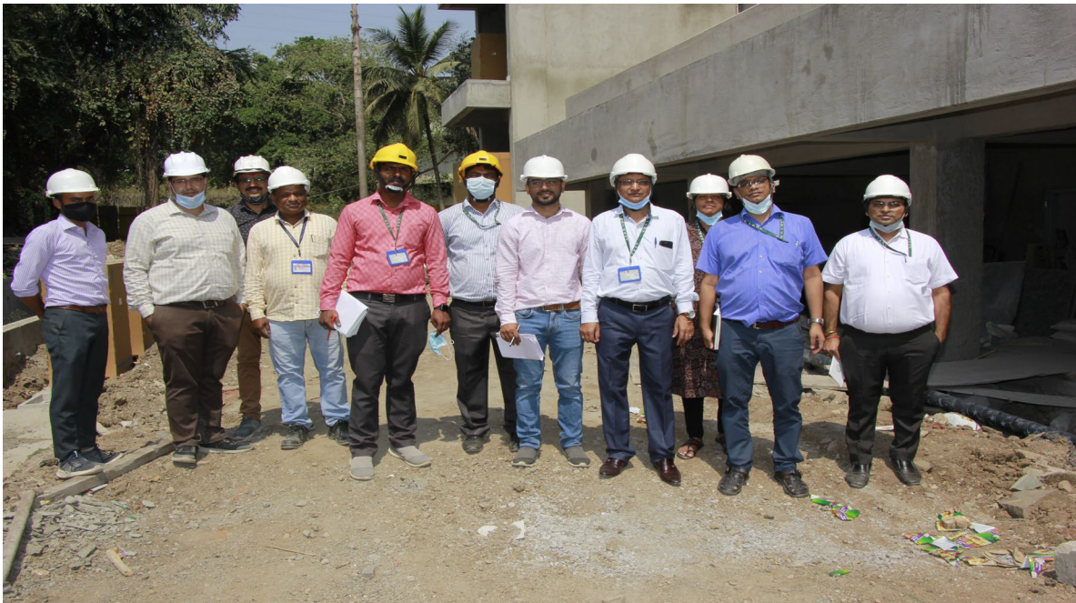
AERB Team inspecting the construction site of Niyamak Bhavan-C during safety inspection of AERB Office premises
